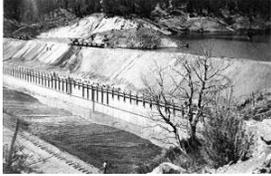
**Little Bear Dam Construction.** Pictured here in 1910 is the new design concrete corewall dam at Little Bear Gorge. Three engines and 45 ore or dump cars were used in the construction that started in 1904.
